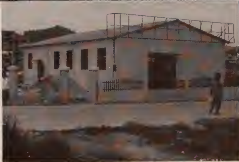
ONE OF MANY NEW CHURCH BUILDINGS IN KOREA, THIS ONE IS PREFABRICATED
